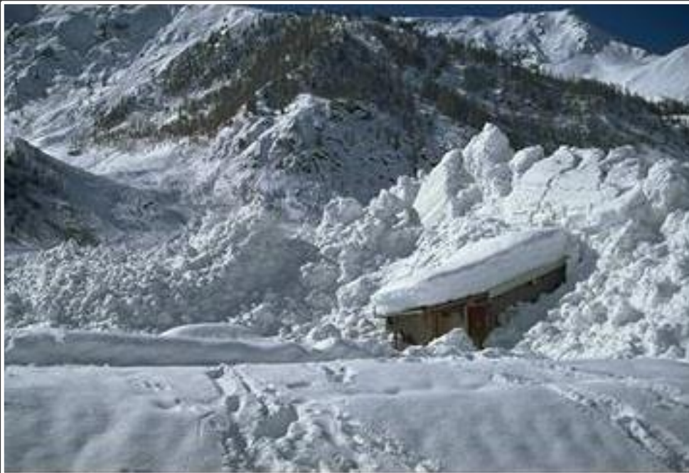
Avalanche deposit on a dwelling house © Irstea ETNA
